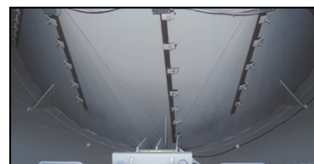
Floating Electric Heat
