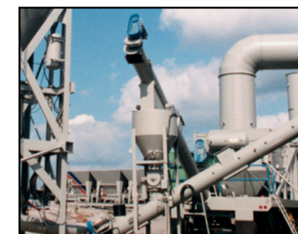
Indian Fines Dust Return System
