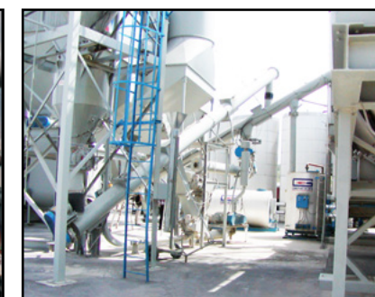
Illinois Fines Dust Return System
