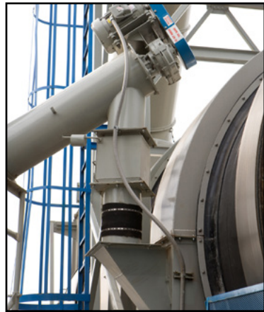
Baghouse Fines Return
