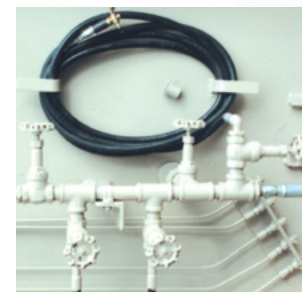
Built-in Spray Clean Out
