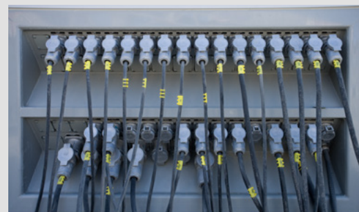
Power Plug Bay
