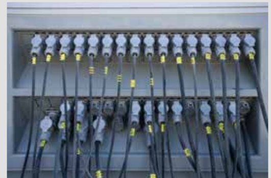
Power Plug Bay
