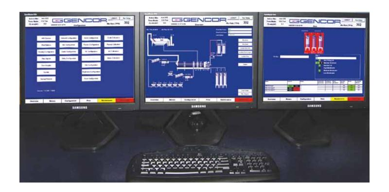
The Gencor Ultralogiks™ Plant Control System's main operating screens display a logical presentation of operating data through the use of segregated screen sections. The upper section displays items at the point of liquid asphalt injection; the center section offers selectable views of motors, maintenance, or event log information as well as configuration settings and calibration screens. Detailed user screens for each equipment component are displayed by simply clicking on the equipment image.
