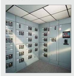
Gencor's control centers offer the ultimate in structural design and efficiency. The center mounted on a heavy steel beam, is a split level design allowing the operator a 360° degree view of the entire plant. The motor control center is situated on the lower level of the unit for operator convenience.
